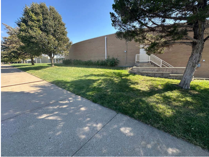
1-019 Remove roof drain and provide new notch in brick parapet for new roof scupper and downspout. See Drawings for locations
