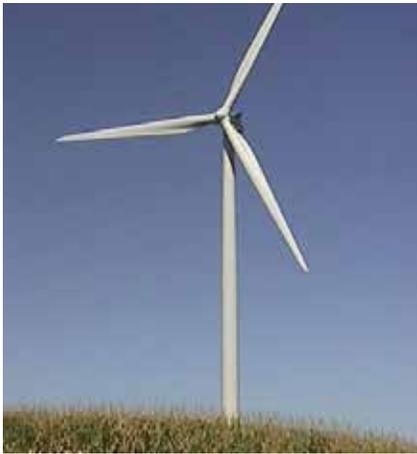
The college installed three turbines on campus in 2008 designed to last 30 years. The free standing towers are 100 feet tall with an additional blade height of 24 feet. The average energy production of PCC's
